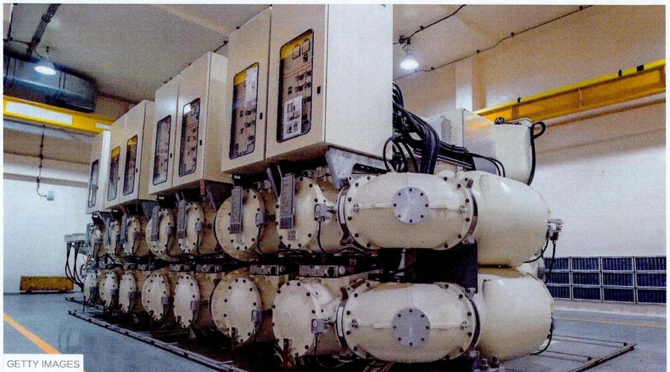
Gas-insulated, high-voltage switchgear almost always uses SF6
